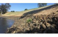
**Scour protection** – Structural bank protection (i.e. rock) armour the underlying sediments and protect them from fluvial and wave action.
