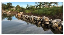
**Figure 25.** Example of rock fillet bench protection in the Kalang River
