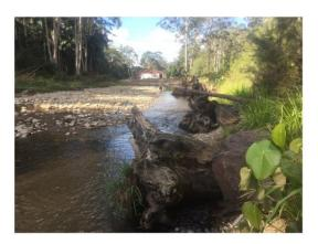
Figure 27. Instream timber toe protection
