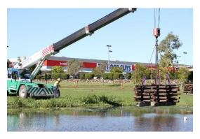
Figure 28. Modular complex timber structures (photo Catchment Solutions)
