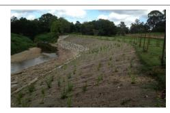
Hydraulic roughness – Structural works provide frictional resistance which dissipates flow energy and reduces the near bank velocity and shear stress. Timber structures have a reduced design life and may not be appropriate for providing long-term protection to high-value
