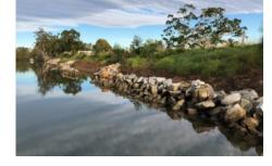
Scour protection – Structural works dissipate the wave energy and protect the bank from wave action.
