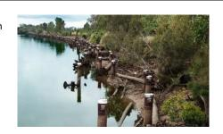
Hydraulic roughness – Structural works provide frictional resistance which dissipates flow energy and reduces the near bank velocity and shear stress. Timber structures have a reduced design life and may not be appropriate for providing long-term protection to high-value built assets.
