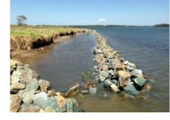
Wave and scour protection -Structural works dissipate the wave energy and protect the bank from wave action.
