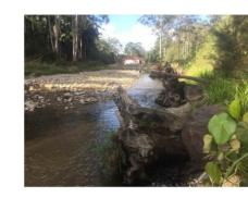
Hydraulic roughness – Structural works provide frictional resistance which dissipates flow energy and reduces the near bank velocity and shear stress. Timber structures have a reduced design life and may not be appropriate for providing long-term protection to high-value built assets.
